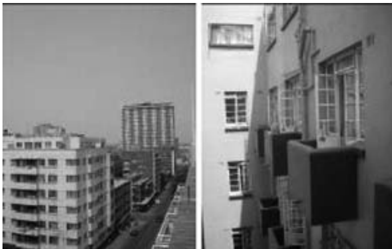
Photos 11 and 12. Buildings Renovated by the Madulamoho Housing Association in the Centre of Johannesburg
